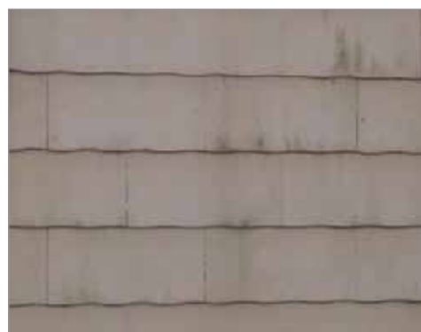
Asbestos-containing shingles
